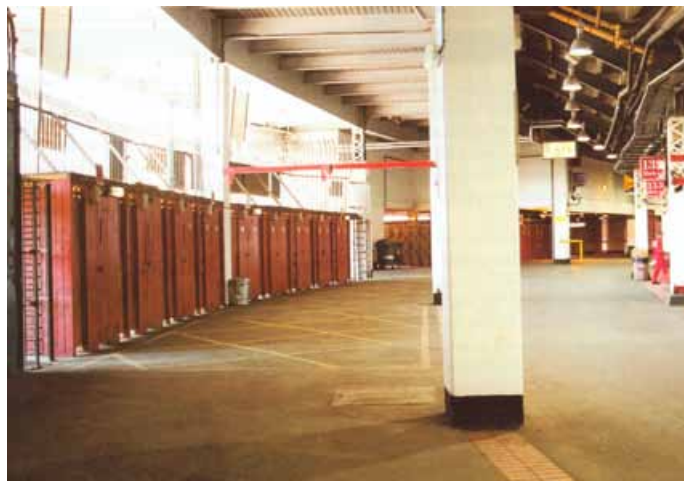
Look for the hazards
